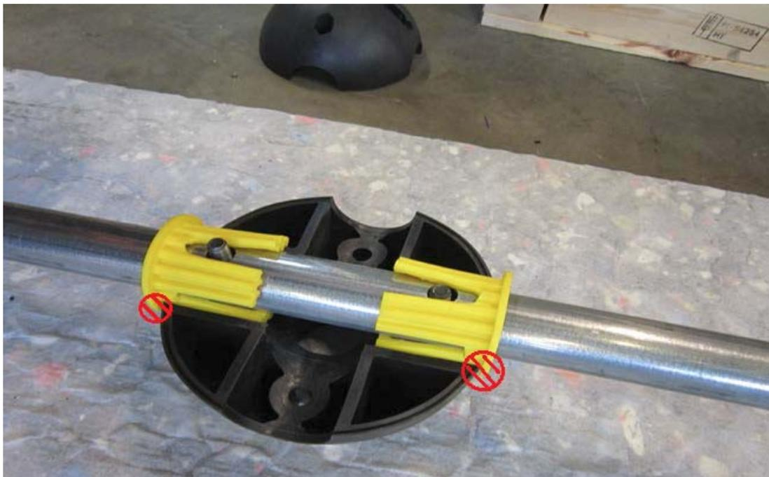
3. Lay the top half on the bottom half and tighten both M10 bolts in turns. The bushings may slide out 1...2mm but not more.
