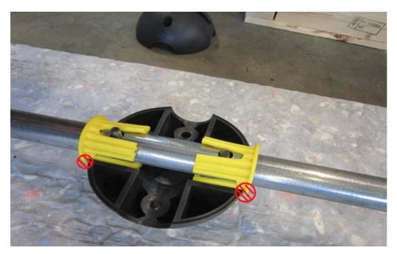
3. Lay the top half on the bottom half and tighten both M10 bolts in turns. The bushings may slide out 1...2mm but not more.
